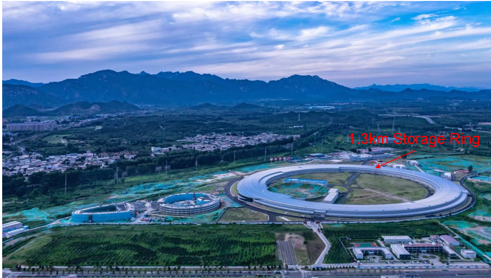
View of HEPS under construction
